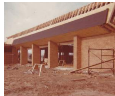
Rox Arena under construction
