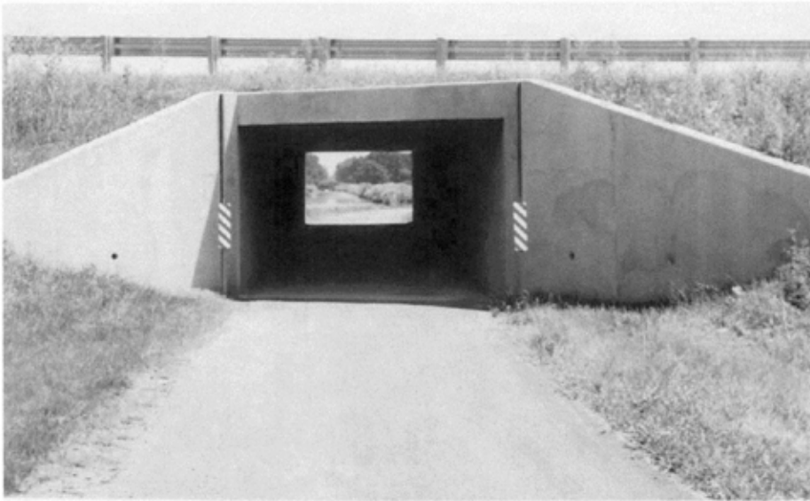
BOX CULVERT INTENDED FOR FUTURE BIKEWAY Figure 17-2AN
