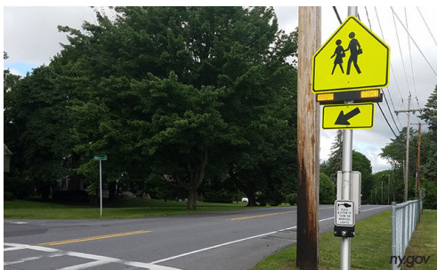
Rectangular rapid flashing beacon
