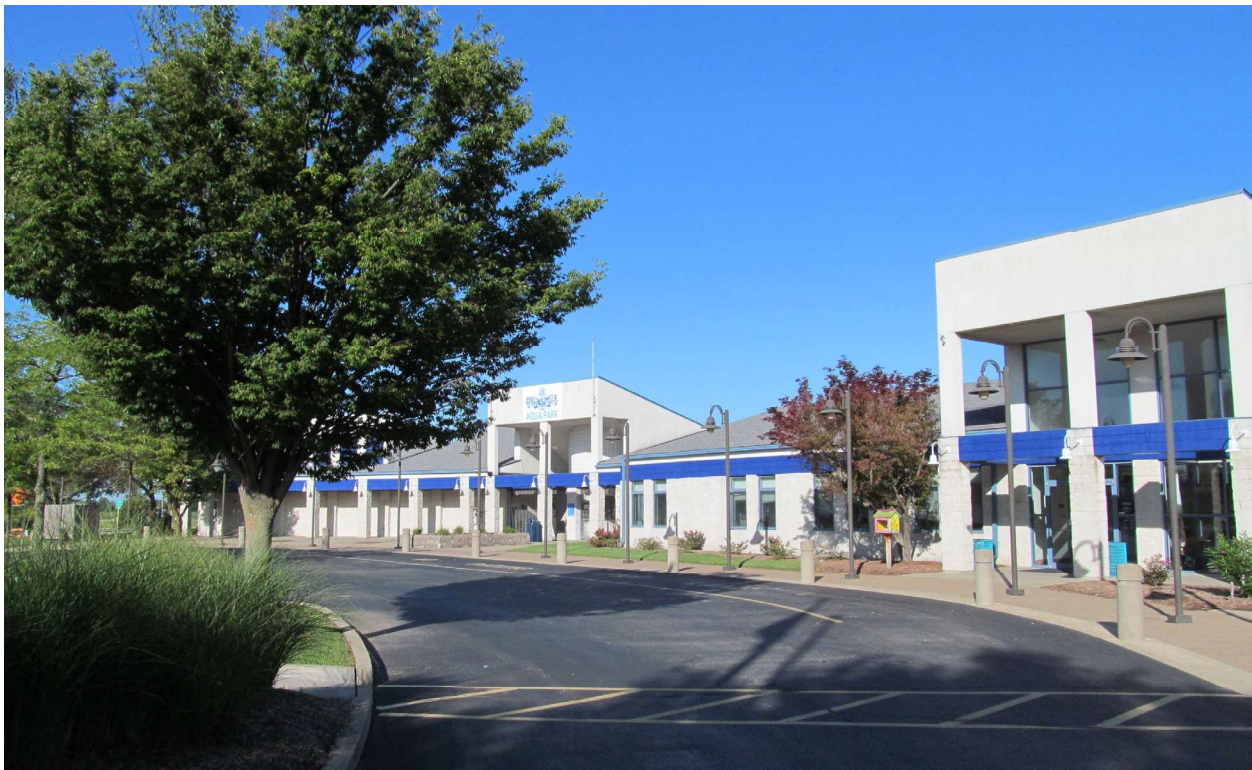
Activity Center front entrance
