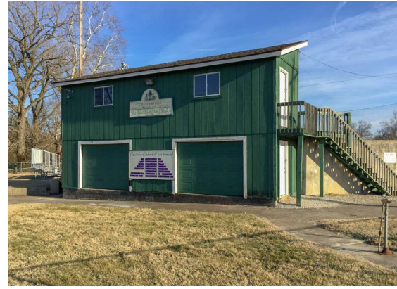
Football concession/press box/storage building
