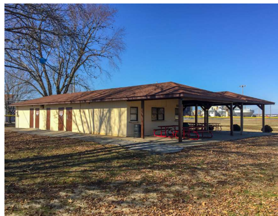
Jaycee concession/restroom needs upgrade/expansion
