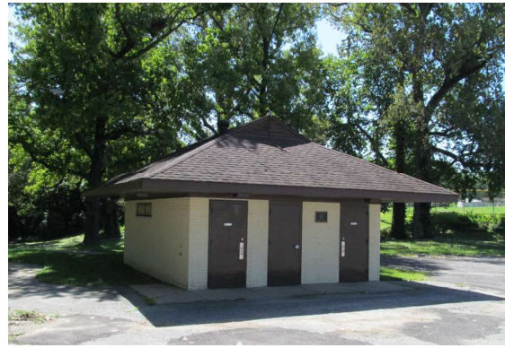
Dated Restroom Facility at Woodland Park
