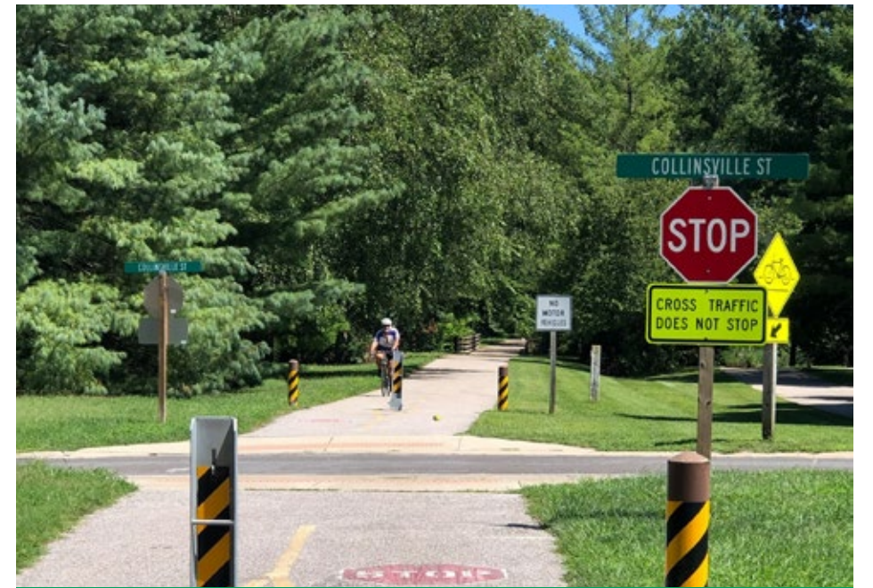
Cyclist traveling along Class-One bikeway with an at-grade crossing.
