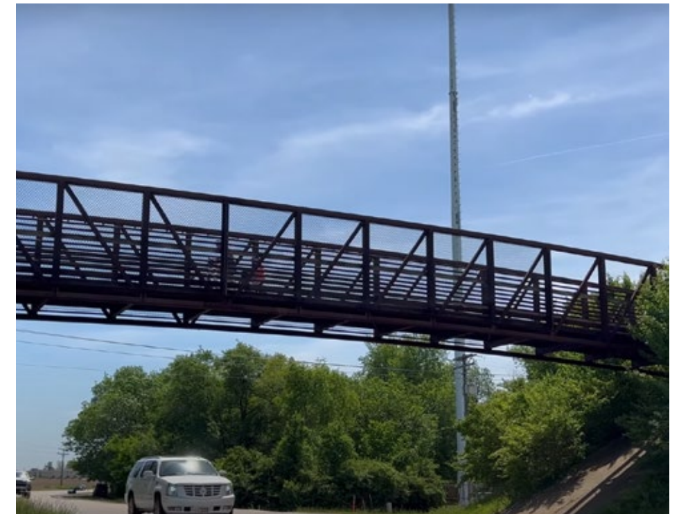
MCT Goshen Trail bike/pedestrian bridge over IL-162
